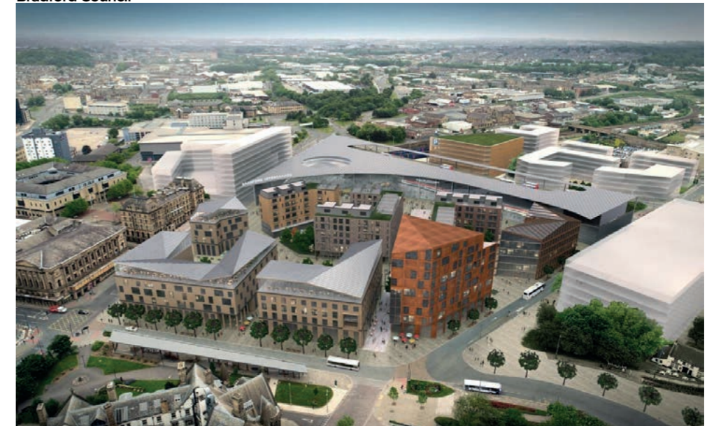
Two computer-generated images of how a future city rail station could look. Images courtesy of Bradford Council
